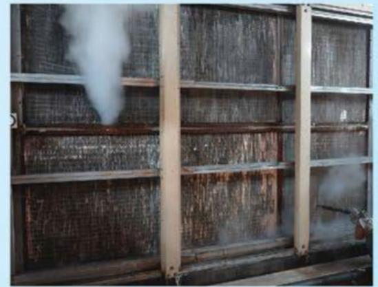
The duration of steam cleaning depends on the level of contaminants, its coil size and depth. Extraction is a gradual process; beginning from the surface and gradually progresses into the inner depths before breaching through.
