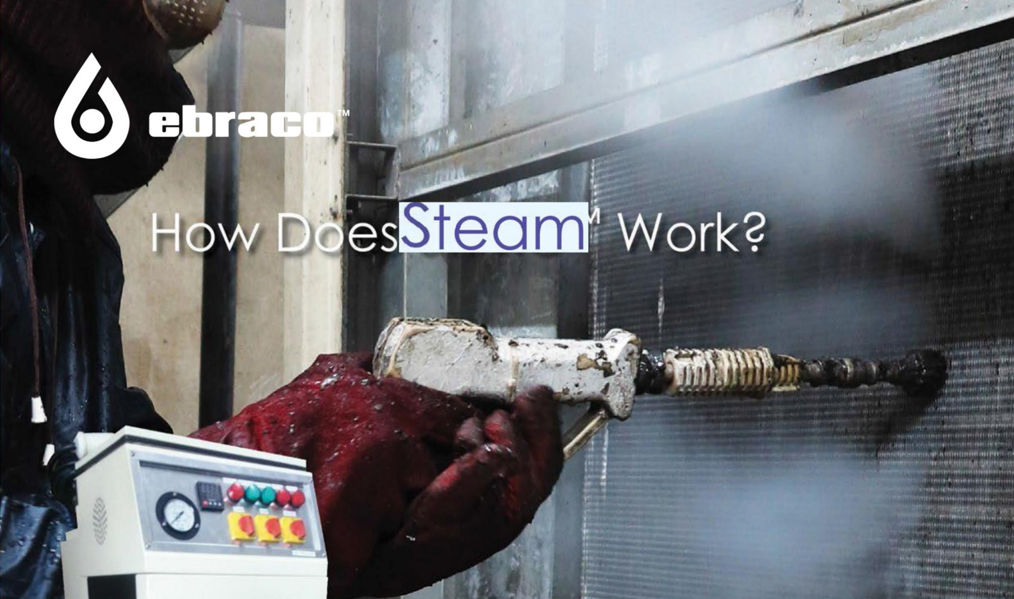
The key to steam cleaning method is heat. It provides thermal shock and boost steam's expansion rate (1500X) to water droplet at a much higher level.
